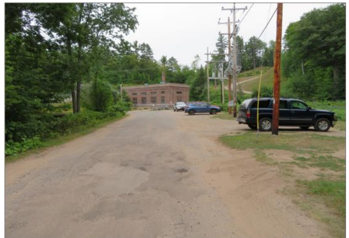
Figure 6: Parking Area for Dead River Gorge Waterfalls and Reany Creek Waterfalls. Note Power Plant Building and Dirt Road Leading to Dead River Gorge in Background. Photo by Dave Adler.
